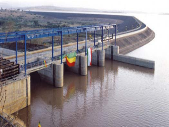
Gilgel Gibe I Hydro Electric Power Dam
