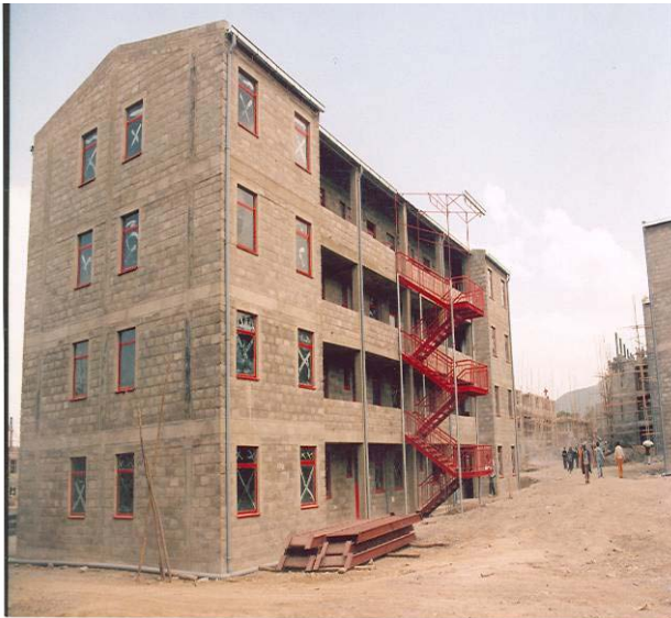
Condominium houses being built by the government
