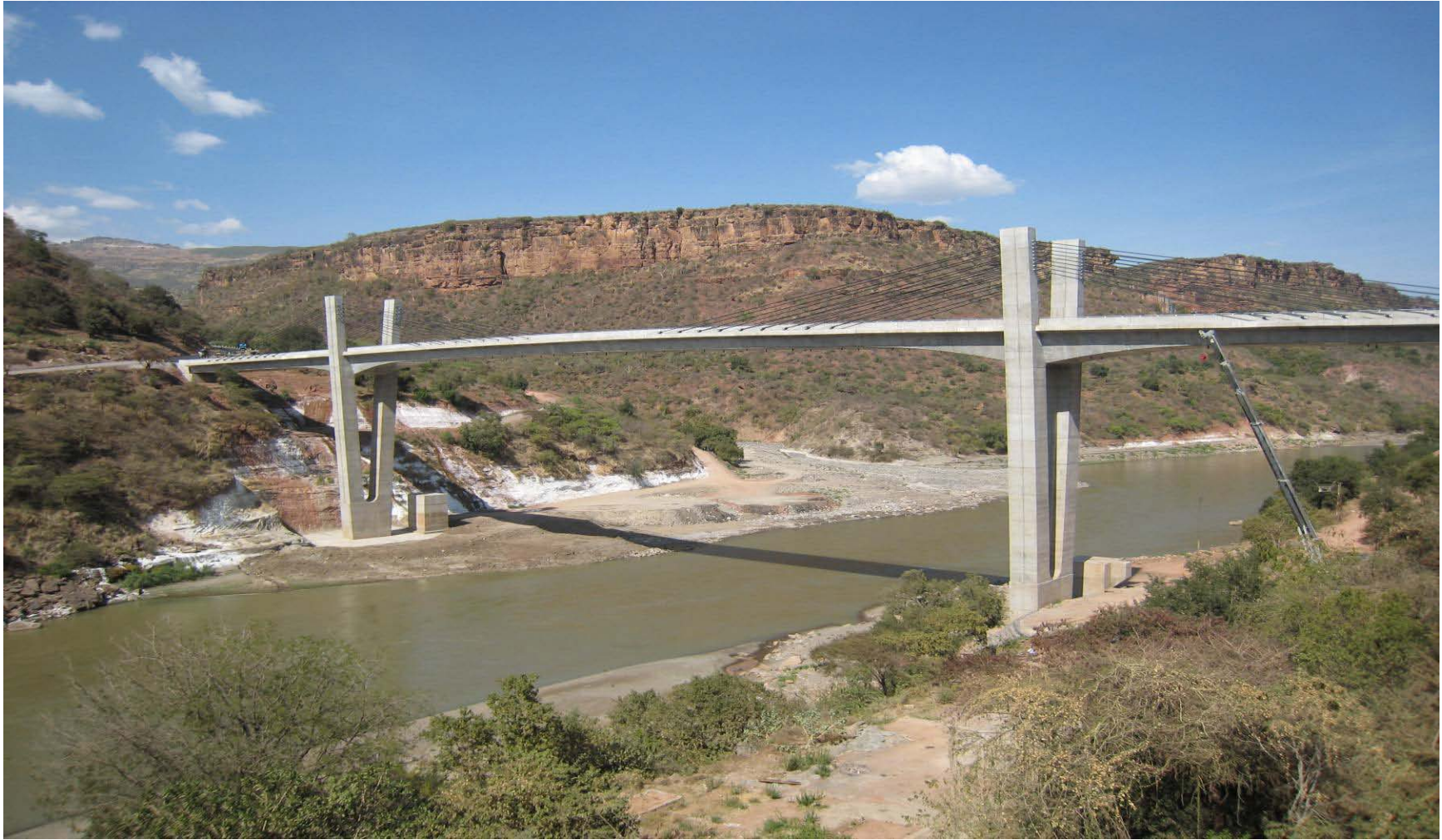
The Addis Ababa-Goha Tsion-Dejen Road Rehabilitation Project which includes the “Renaissance Bridge” over the Abay Gorge constructed with Japanese grant assistance
